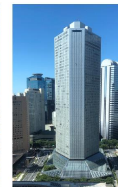
Shinjuku Sumitomo Building (Completion: Mar 1977, Renovated: Jun 2020)
